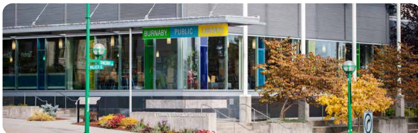
Tommy Douglas Library makes use of a geothermal heating system, which results in very low greenhouse gas emissions intensity.
