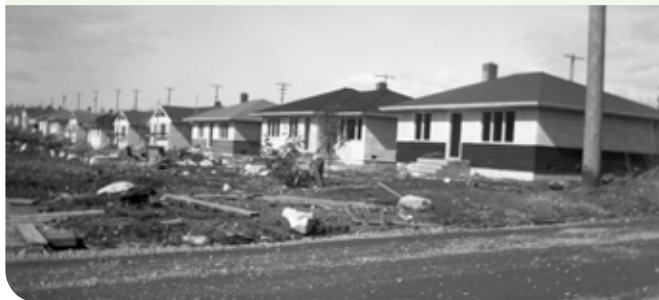
Suburban houses under construction in Willingdon Heights in 1947. City of Burnaby Archives 010-032
